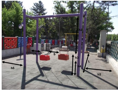
Figure 2. According to TS EN-1176-2 (2010), symbols of safety criteria for swing (Orjinal, 2013)
