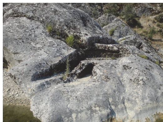
Fig. 18) Western footing of the wooden bridge
