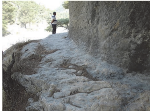
Fig. 13) A rock-cut section of the road on the eastern bank of the Myros River.
