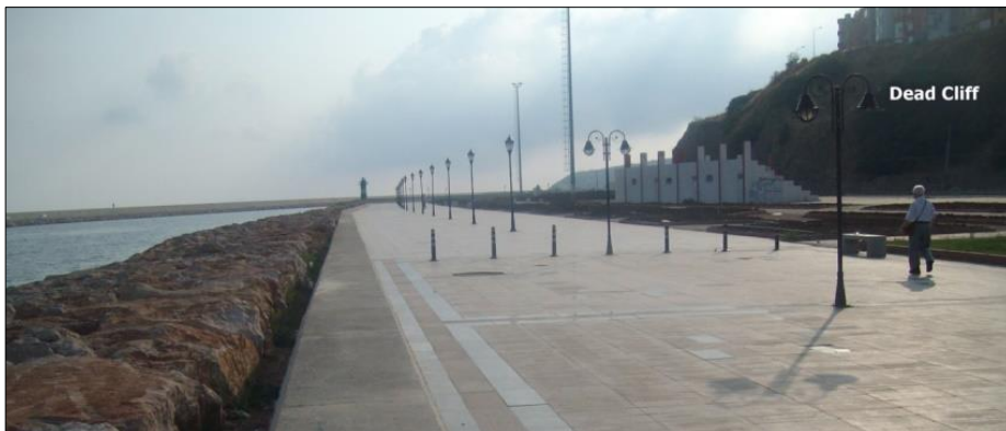
Photo 5: Coastal Landfills that Serve to the People of Bandırma as a Walking Area (2013).
