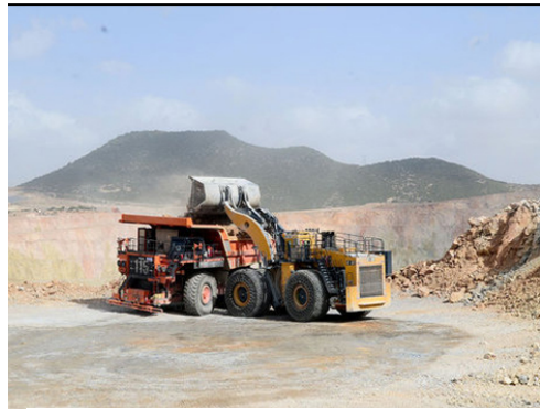
Figure 1 L-1350 is loading to Hitachi HT-AC-5500 OHT at the gold mine in Uşak
