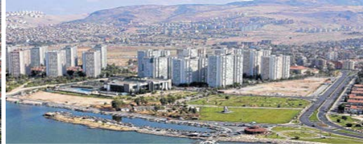
Figure 6; View from Mavişehir work area
