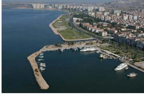
Figure 3; View from work area
