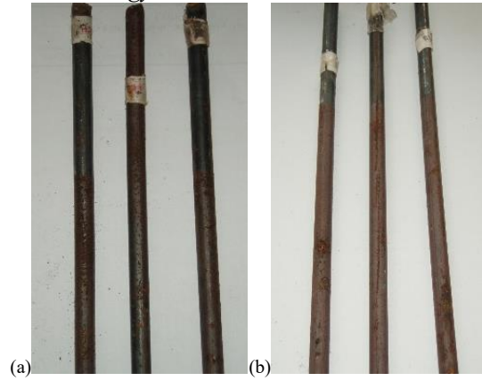
Fig. 14 Corrosion activity of reinforcing bars (a) M1Cl, (b) M2Cl
