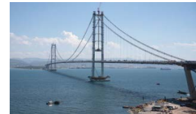
http://t24.com.tr d) Osmangazi Bridge in the Gulf of Kocaeli
