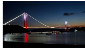
http://www.mavikocaeli.com.tr c) Yavuz Sultan Selim Bridge
