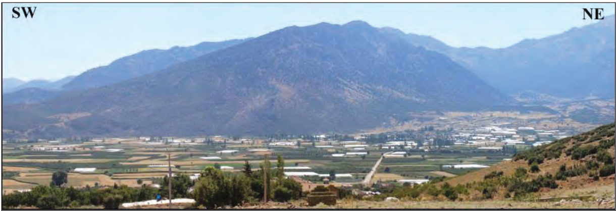
Figure 13- General view of Salur fault (looking to NW).
