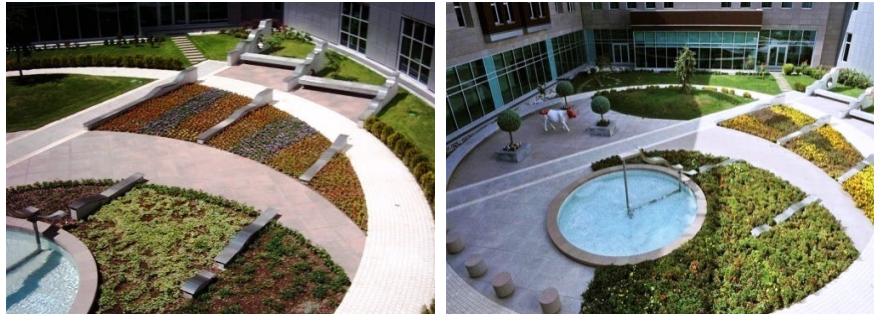
Visual 10. Mesa Hospital Building (Beyhan & Erbas, 2013)
