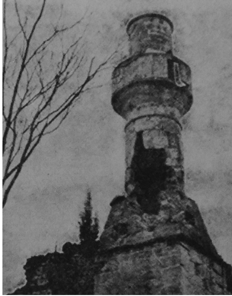
Figure 4. Minaret of Şehzâde Süleyman Paşa Mosque at Bolayır, damaged by gun-fire from HMS Queen Elizabeth on March 29th, 1915 (Photo: Harp Mecmuası 5, 1915, 76).
