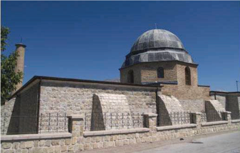
Fig.9b: Malatya, Great Mosque, exterior, south Wall
