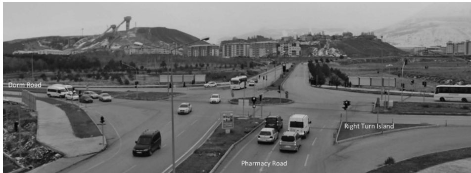
Figure 9. Right Turn Island for Pharmacy to West Road Route And Signalization Application
