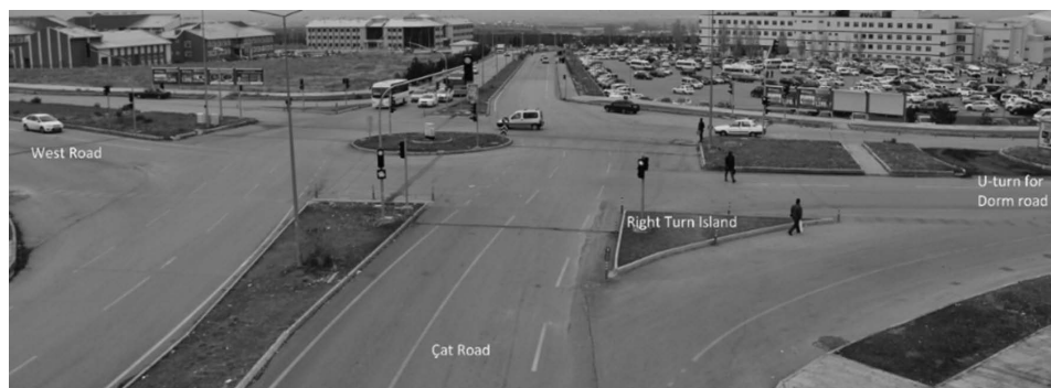
Figure 10. Right turn island for Çat to Dorm Road route and U-turn for Dorm Road
