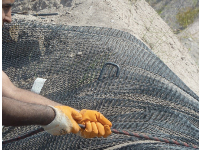
Figure 5. Laying of Tieback Anchors
