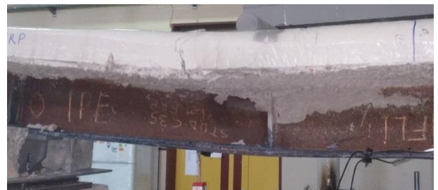
Figure 20. Concrete crushing and deflection of CBW3CFRP sample
