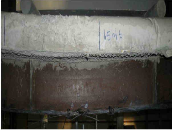
Figure 16. Shear cracks near the loading point
