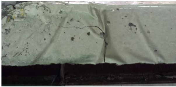
Figure 12. Shear cracks of the CW0CFRP sample
