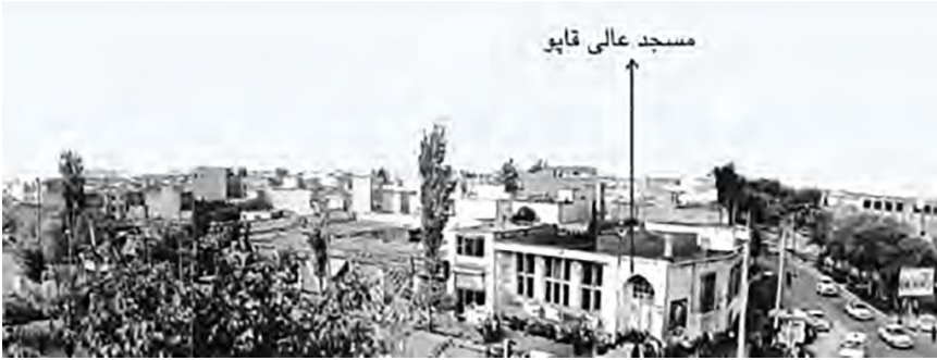
Figure 4. The Destroyed Mosque in Āli Qāpu (Rezazadeh & Peighami, 2013).
