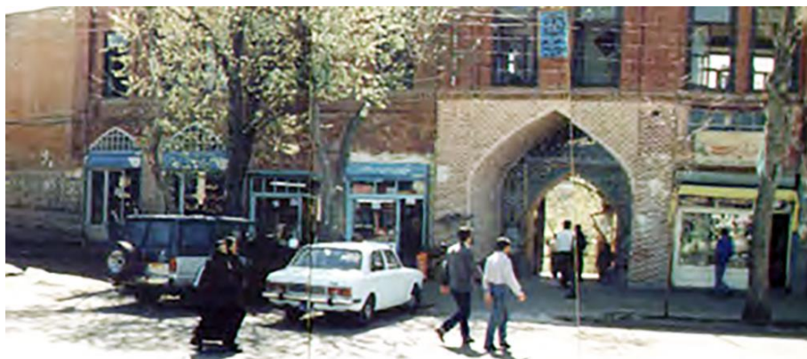
Figure 8. The destroyed old main entrance to the Ensemble (Rezazadeh & Peighami, 2013)
