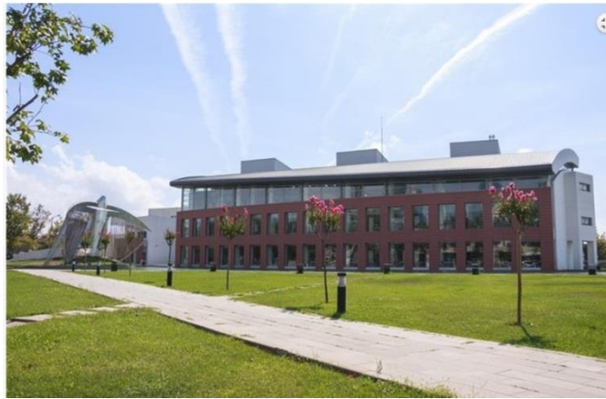
Figure 11. The road across the library was paved and warmed up in the summer. The rainwater there was not able to mix with the soil in this part before. With the infrastructure and landscaping in this region, the area has become a more livable area.
