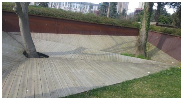
Figure 13. The Material Used In This Structure Was Not Colored. So, Over The Time, The Corten Is Washed Up Into The Soil And Afford The Necessary Fertilization Of The Soil.
