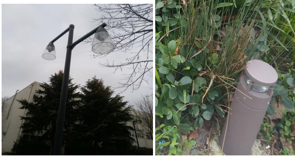
Figure 16. LED Light Bulbs In ITU Campus
