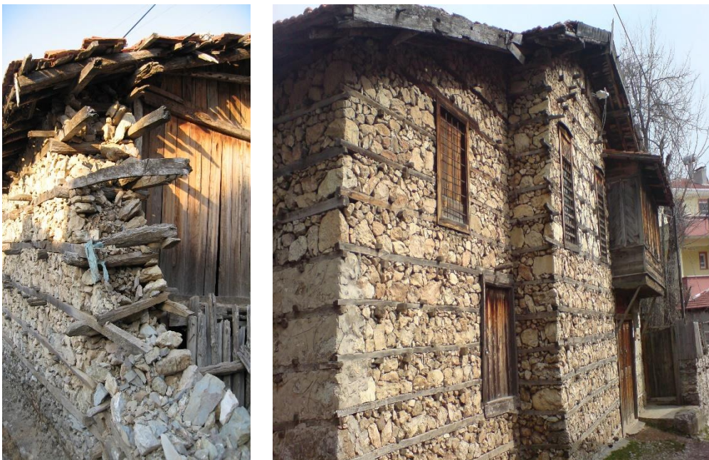
Figure 6. Düğmeli Duvar- Butted Wall (Çelik 2008)
