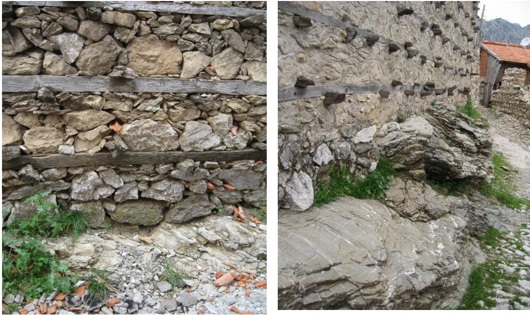
Figure 4. Foundation of the Buildings (Çelik, 2009)
