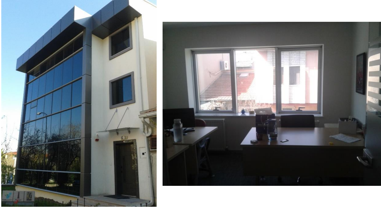
Figure 2 At left Building 1 exterior picture that examinations were mainly went on. Photo was shot at 21st April, 2015. At right, an interior image of Building 1 showing the exterior walls adjacent to the curtain wall. The photo was shot at 27th April, 2015.
