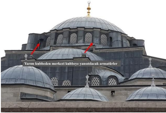
Fig. 13. The central dome and north half dome.
