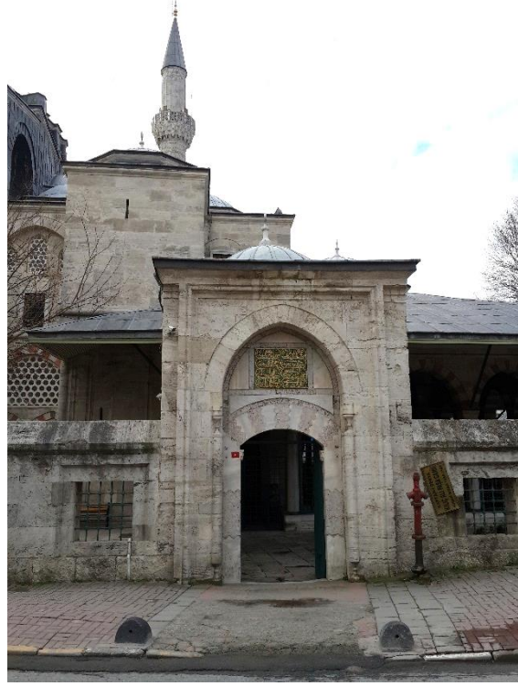
Fig. 6. Eastern entrance of the courtyard.
