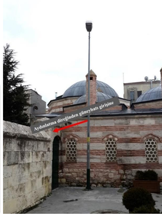
Fig. 8. Southwest corner of the courtyard.
