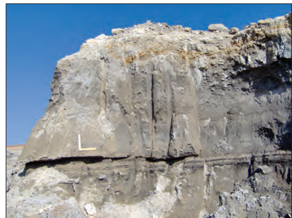
Figure 8-General view of the H4 landslide
