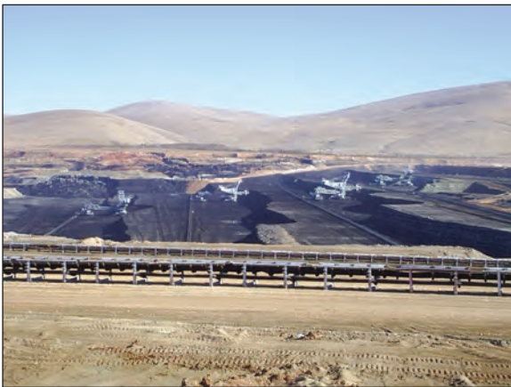
Figure 6- A large landslide (H3) developed in the permanent east slope
