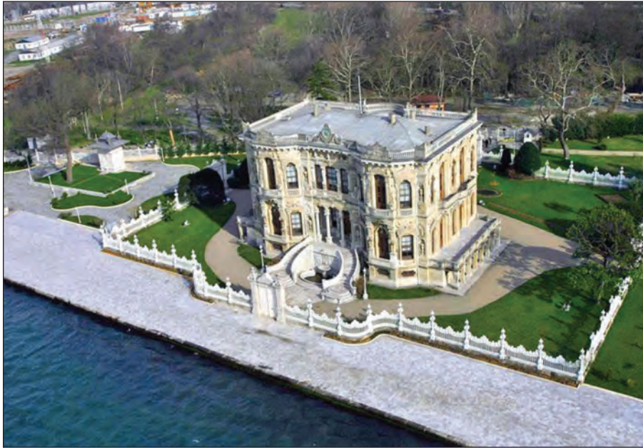
Figure 1- View of Küçüksu Palace (looking east) (www.millisaraylar.gov.tr).
