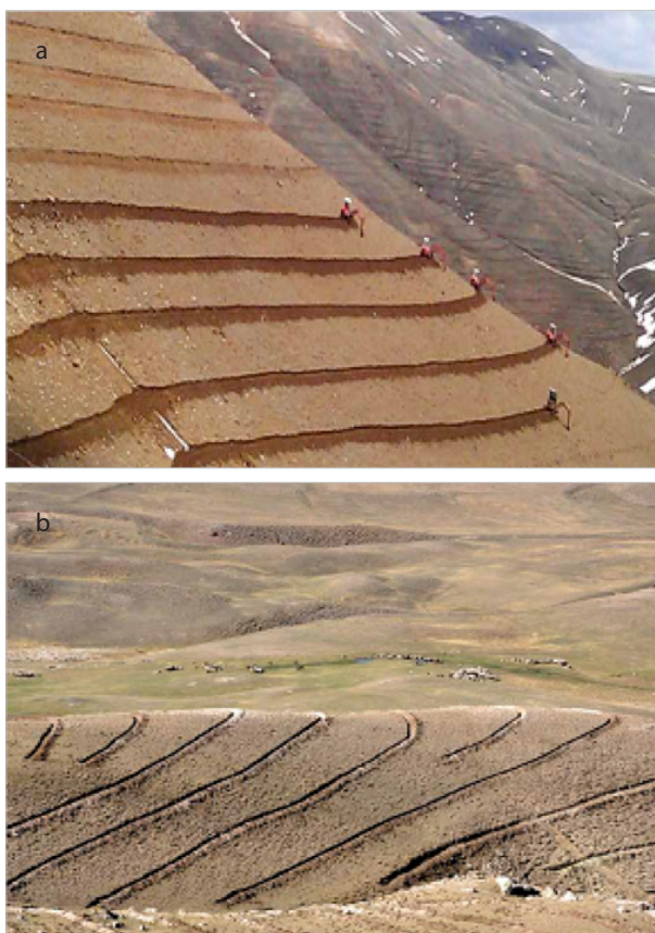
Figure 8. a, b. Contour terracing for erosion control (a) and improving soil moisture recharge and forage production (b) (GDCDE, 2015)
