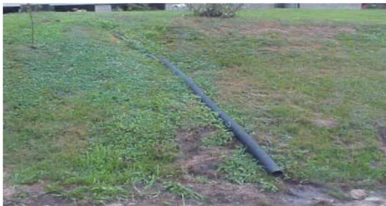
*Figure 2.* A typical straight pipe discharge (EPA Region 4, 2002).
