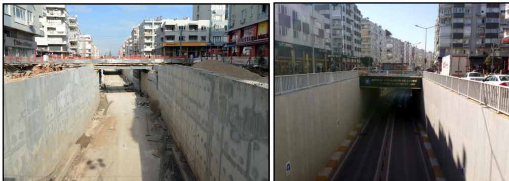
Figure 3. Construction (Gorez 2017) and present state of underpass for vehicle.
