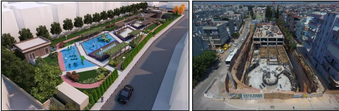
Figure 5. Construction of underground car park planned in Göçmen Park (Antalya Metropolitan Municipality 2018).
