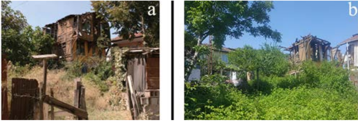
Figure 8: The heavily damaged building (a) was partially lost in 2018 (b).
