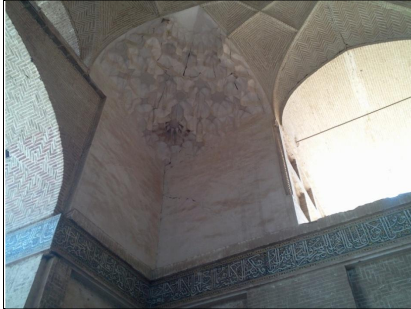
Figure 7. An overview of the great gaps created in the beautiful Moqamas of the mosque and above the Mihrab (Photo: Author)
