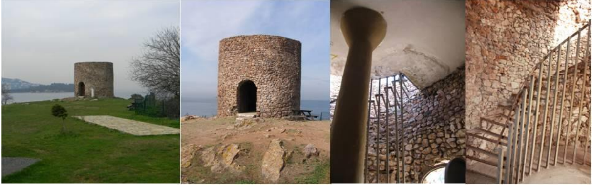
Figure 2 Current state of the mill (Kıraç,B., Töre,T., 2014)
