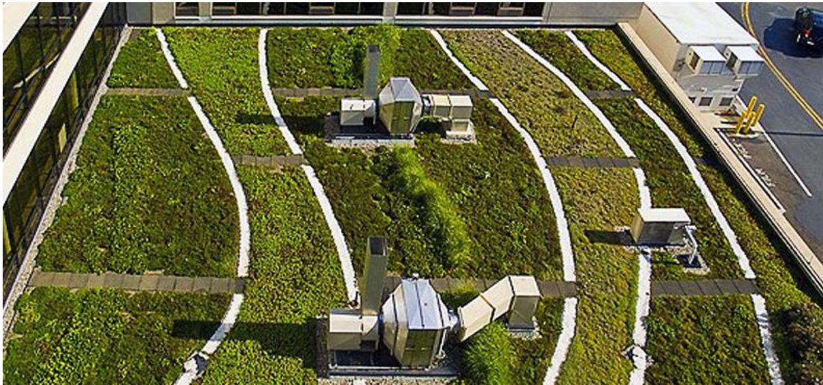
Figure 3. ICU Rooftop Garden. Example of extensive roof garden (URL 5).
