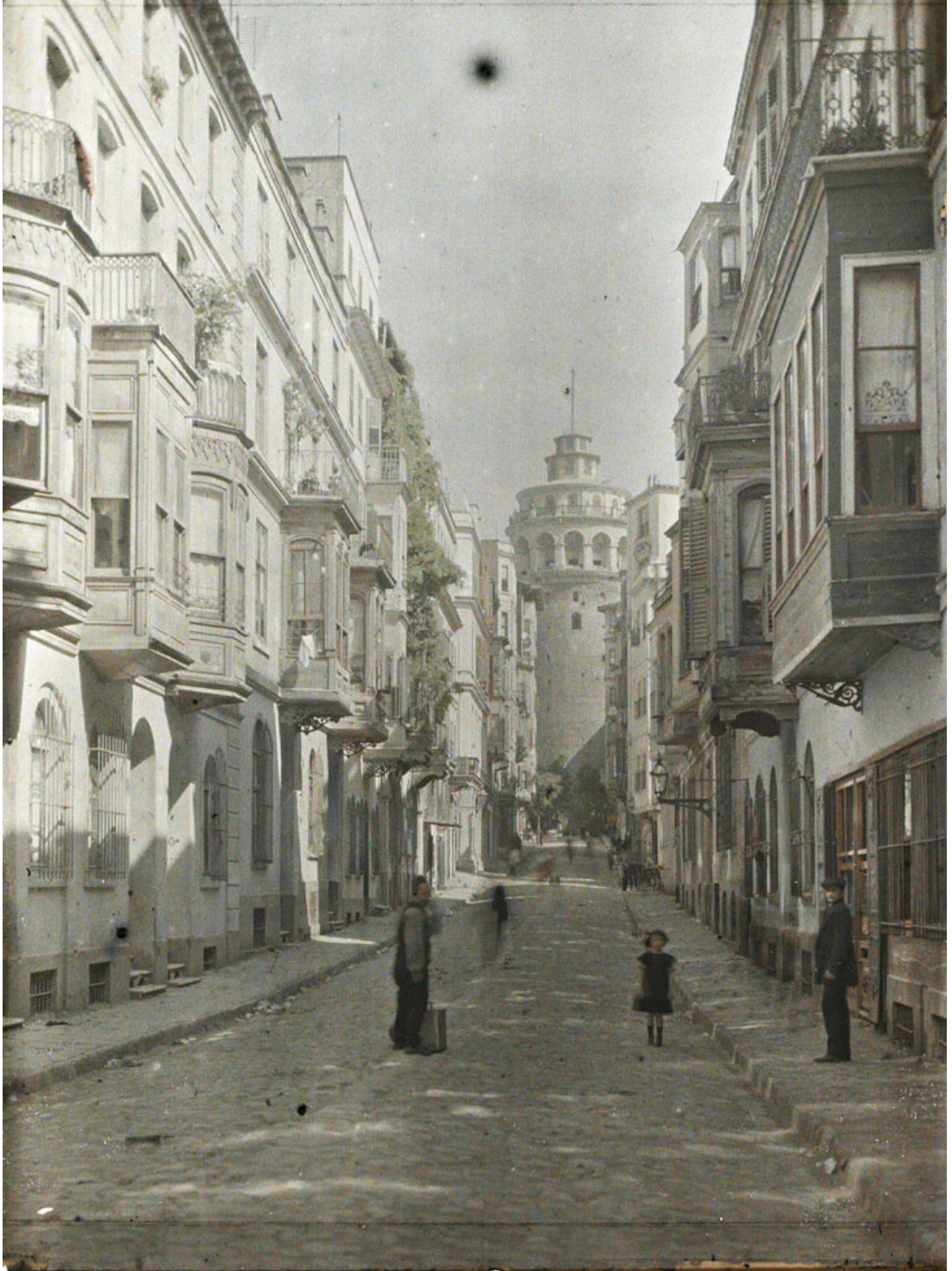
Figure 5. New row of apartments built after the demolition of Galata walls.
