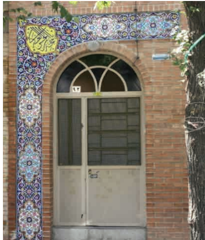
Fig. 4. The use of vertical diagonal framing in the entrance view of a house built in Khakshenasi ST. in the Pahlavi era (Photo by Dordaneh Mohammadi, 2016)
