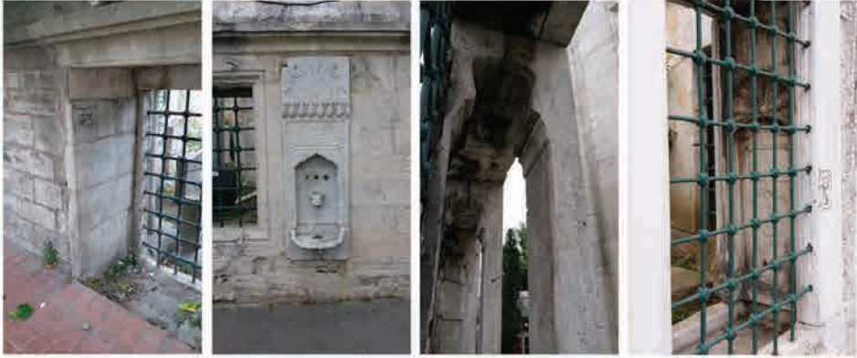
F. 3. The window details of Şehzade Mehmed Mosque; a) Safiye Sultan window sebil , b) twins fountains, c) the arcades in the wall thickness of the quadruple windows, d) Gevher Sultan window sebil (Author, 2018)
