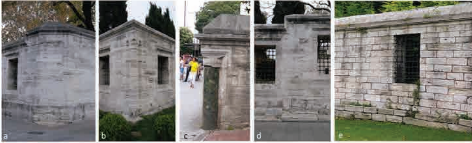
F. 5. The corner turns ( çal köşe ); a, b) Süleymaniye Mosque, c) Şehzade Mehmed Mosque, and the wall base ( duvar pabucu ); d) Süleymaniye Mosque' west surrounding wall, e) Şehzade Mehmed Mosque's north surrounding wall (Author, 2018)
