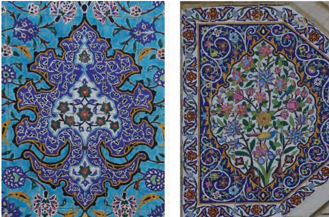
Fig. 10. The use of medallion in Haft rang tile frames made in Shiraz (on the right) and Isfahan (on the left)
