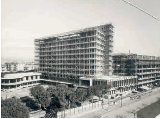
F.14. The Grand Efes Hotel's construction (Kenan Kurtkaya Archive)
