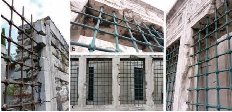
F. 12. Connection details of iron grilles with jambs; a) Kara Ahmed Pasha Mosque, b-d) Şehzade Mehmed Mosque (Author, 2018)
