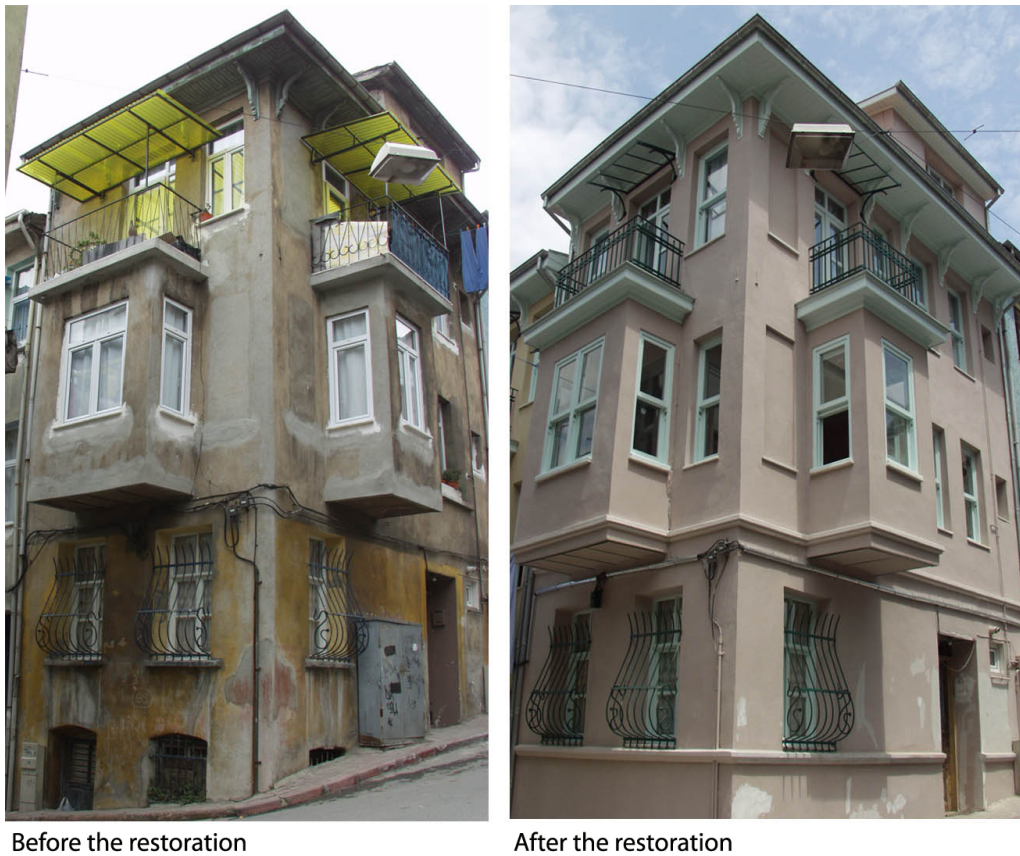
Photo 3. Fener Balat Rehabilitation Project (URL-4, 2011)
