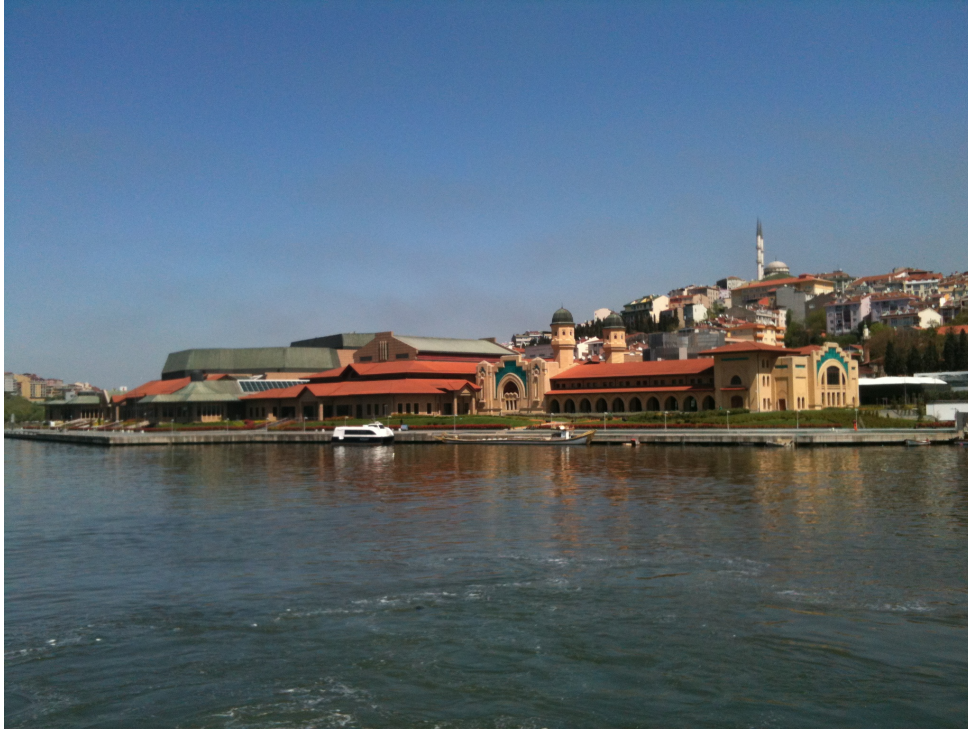
Photo 2. Sütluce Congress Centre (The archive of Eyüp Municipality, 2011)
