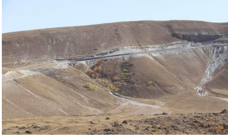
Figure 4. The View Of The New Road In Nemrut Caldera Nature Monument From The Direction Of Tatvan (2017)
