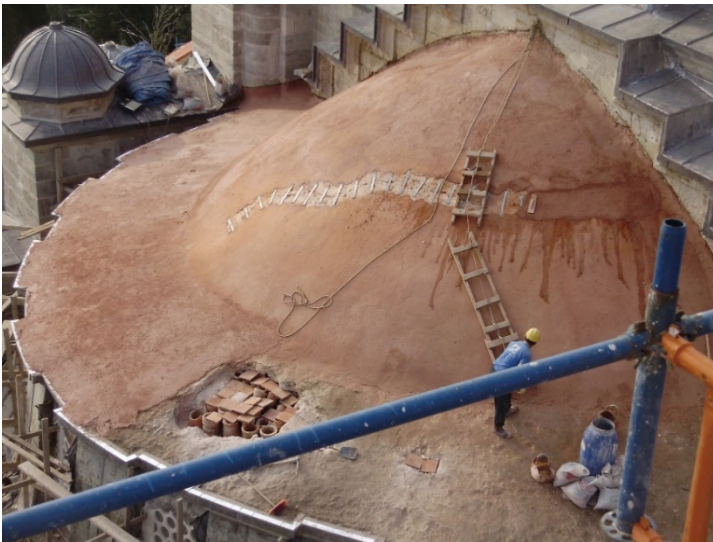
Fig. 4b - Side dome view around the station 4 from outside [34]
