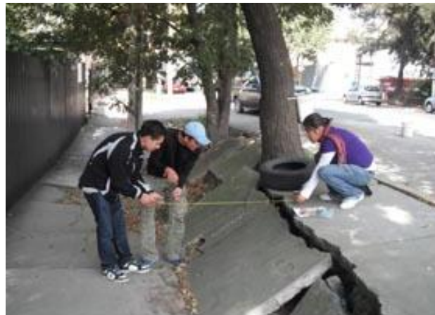
Figure 2. Surface deformation in Mexico City area (The Geodesy Lab)
