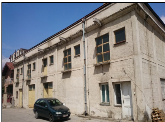
Figure 2. Previous condition of the building (exterior) a
