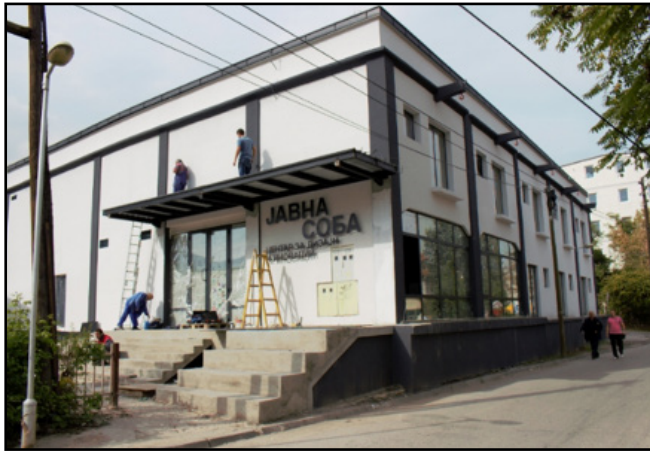
Figure 6. The new condition of the military building after the reuse project and seating area in the courtyard a
