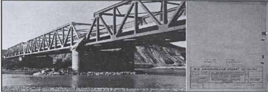
Figure 4.32 Right: Cover page of the project signed by the Department of State Railroads. Left: Genç Bridge in 1952. Source: Unclassified documents from the State National Archives-Republican Archives, KGM Fund, Binder no: 2939; KGM Archives, off-track bridge files, region 8.
