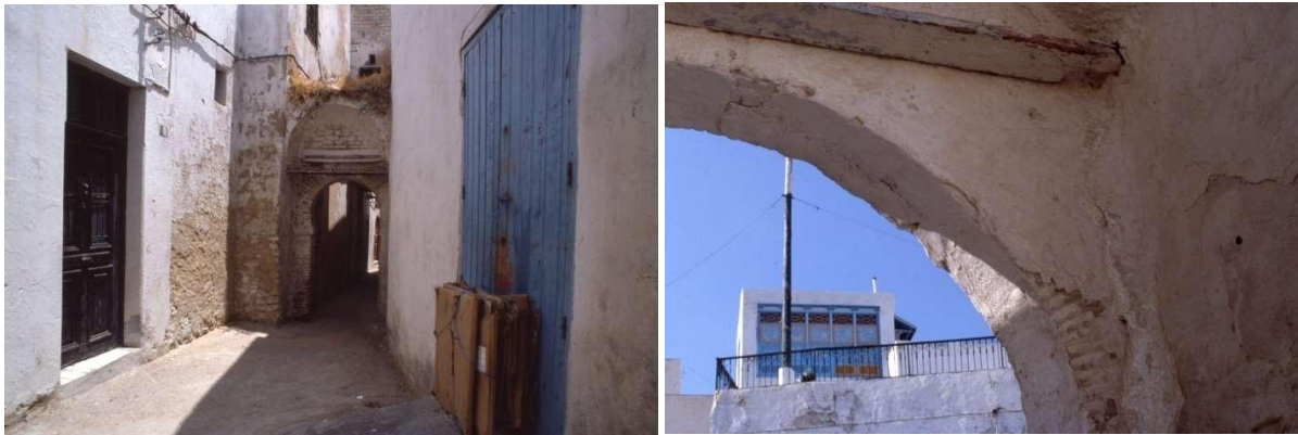
Figure 3. (Left) The location a gate of a dead-end street in the city of Tunis that was demolished Figure 4. (Right) The wooden frame of a gate of a squire in Sidi Bu Said in Tunis. Notice the whole in the corner of the wooden beam to support the gate in Figure 3 and Figure 4
