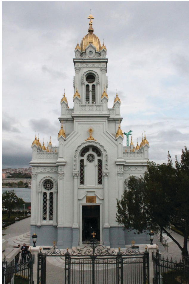
Figure 1. Western façade of church after finishing restoration in 2018. Photographer Blagovesta Ivanova.
