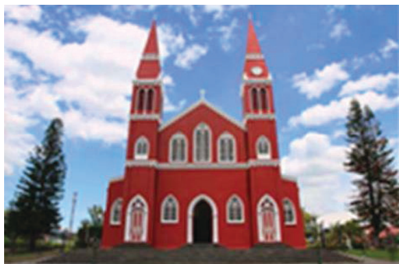
Figure 11. Western façade of the „Iglesia de la Nuestra Señora de las Mercedes“ in Grecia, Costa Rica. http://www.blackincostarica.com/2016/03/our-new-house-in-grecia-costa-rica.html
