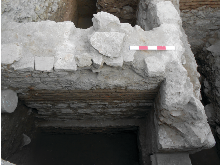
Fig.20: Wall built of stone blocks in regular rows and horizontally placed bricks.
