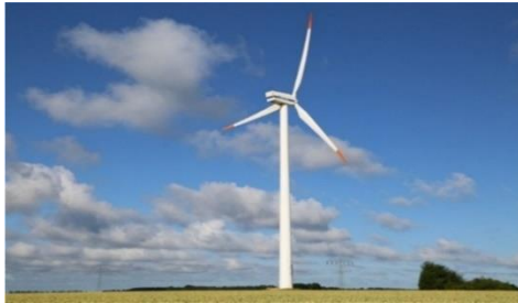
Fig. 5. 1.5 MW wind turbine (“Wind turbine model”, 2019).
