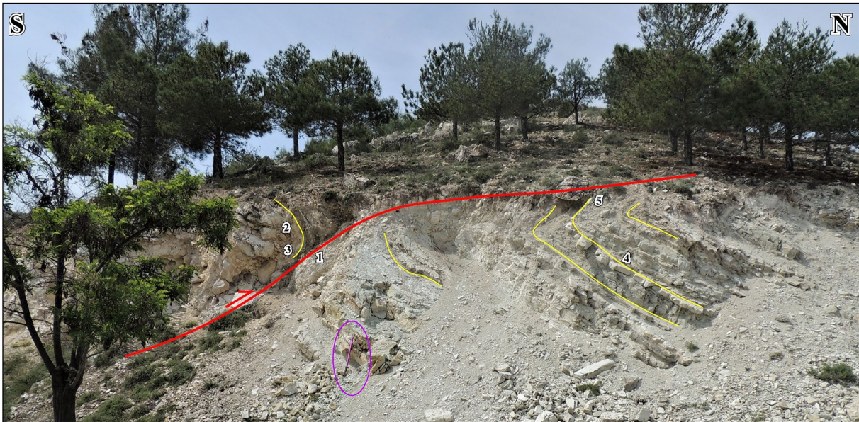
Figure 8-b) The Davutoğlan Back Thrust. The hanging wall has moved northward as drag folds show. The horizontal fold axis has E-W direction. (1) Fault plane: N 60 E, 35 SE; (2) Bedding: N 65 E, 65 NW; (3) Overturned bedding: N 30 E, 65 SE; (4) Bedding: E-W, 40N; (5) Overturned bedding: E-W, 55S.
