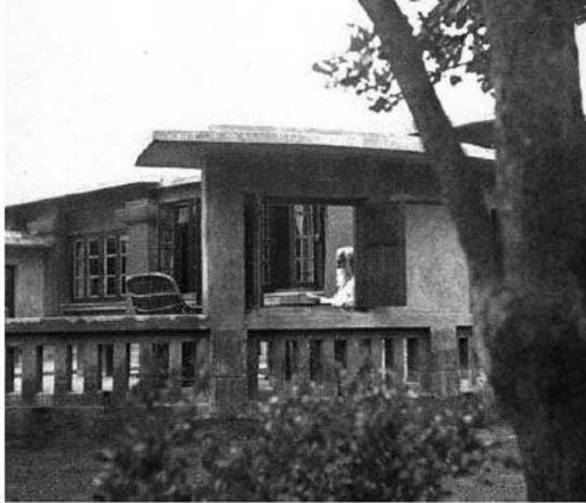
Figure 6. Punascha was Tagore's favorite leisure building, Rabindra Bhavana, archives of Shantiniketan; a photo by Saha, taken in 1930 (Sanyal, 2015: 603)
