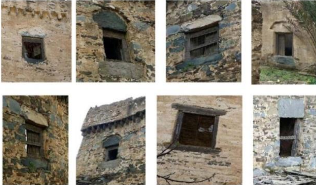
Figure 4. style of windows used in Al Baha buildings (2018)
