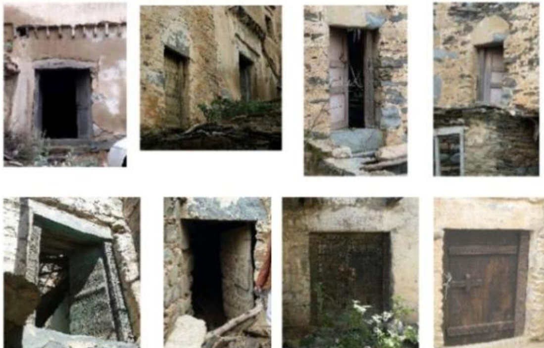
Figure 5. style of doors used in Al Baha buildings (2018)
