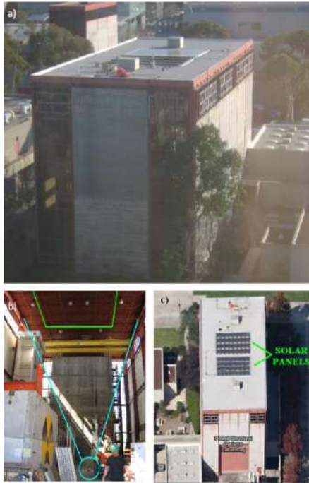
Figure 24 (a) Photograph of Powell Structural Systems Laboratory (PoSL) at the University of California, facing South, (b) photograph of PoSL from inside facing North, (c) Google Earth image of PoSL (north is up) [63]
