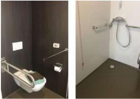
Figure 4. Senior Assist Londerzeel Nursing Home Wet Area Photos
