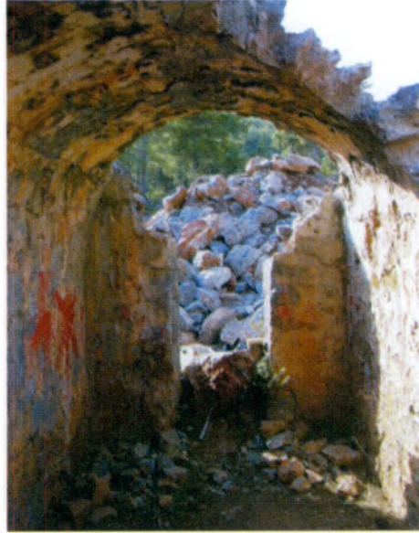
Fig.3 - Internal view (from east to west)
