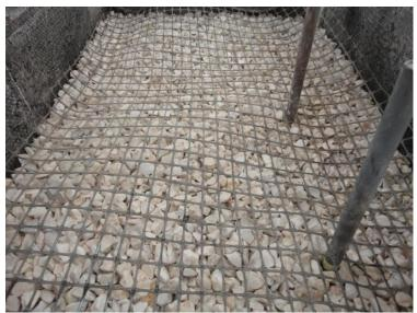
Figure 10. Placing the geogrid.
