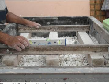
Figure 11. Placing and leveling the track panel.
