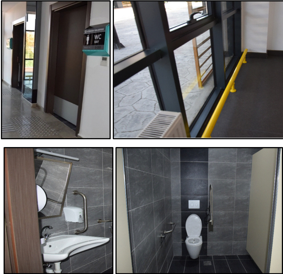
Figure 2. Door protective plates, disabled barriers and restroom samples (Original, 2018)
