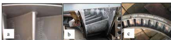
Figure 11. Visual inspection of 1st stage turbine nozzle (a) before operated (b) after operated by HSD taken on Major Overhaul (c) after operated with B5 for 1 month
