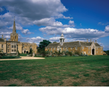
Nevill Holt Opera Theatre Facade (Photography: H el ene Binet, architecture.com)
