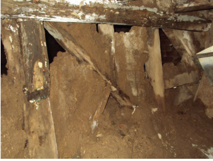
F. 19: Timber Structural Elements on the Intermediate Wall in the Basement Floor (It can be observed because of the plaster fall) (PA/18. 11. 2009)
