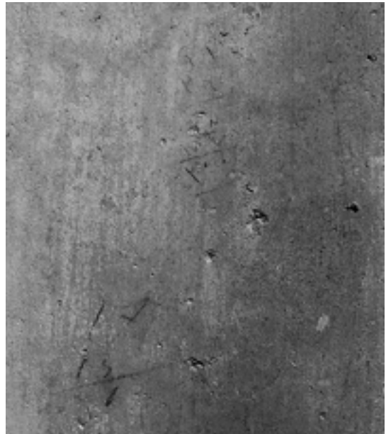
FIG. 9 Records written in Ottoman Turkish on the front face of the left side of the door frame of the entrance to the Yenikapı Hamamı (Bathhouse).
