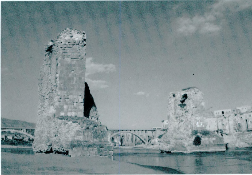
Fig. 15 — Hasan Keyf bridge.
