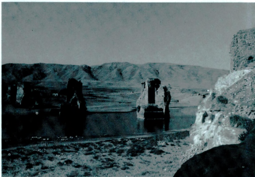
Fig. 13 — Hasan Keyf bridge.
