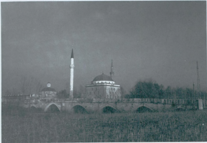
Fig. 24 — Yeni İmaret (Bayezıt) bridge.
