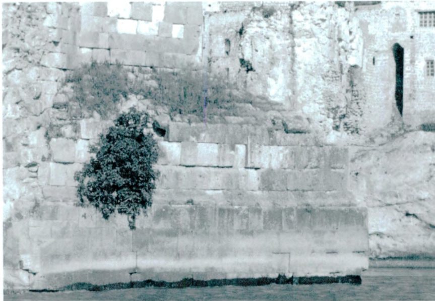
Fig. 16 — Hasan Keyf bridge.
