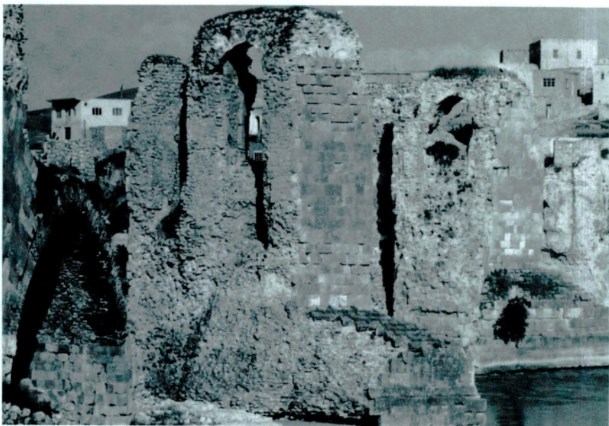
Fig. 14 — Hasan Keyf bridge.
