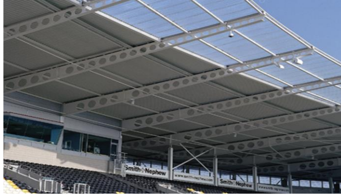
Figure 1: Roof support beams [18].
